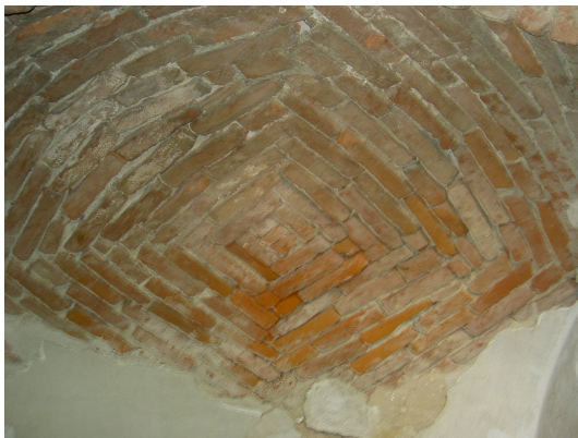
Figure 3. Brick masonry vault.
