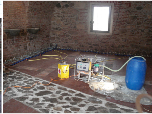
Figure 8. The used grouting equipment
