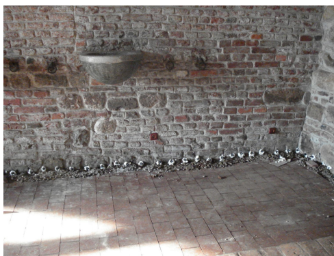
Figure 6. Put and stuffing the tubes
